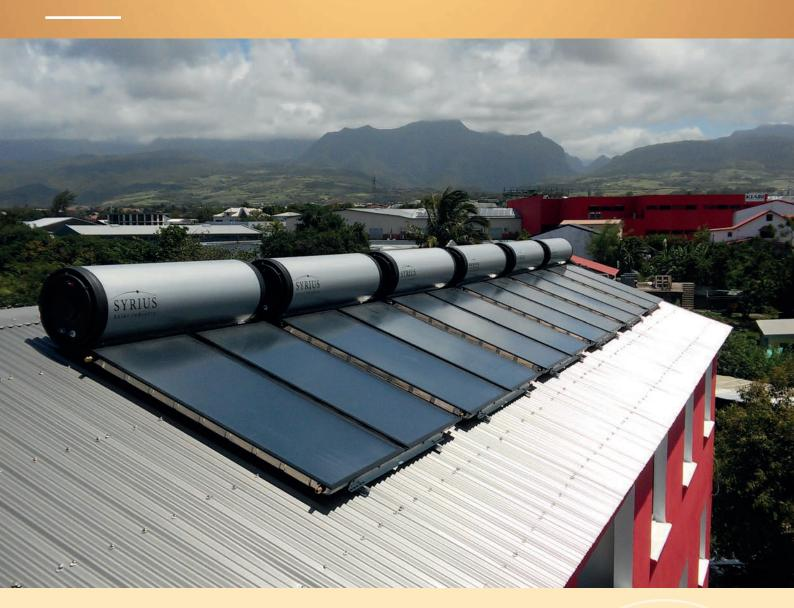
The solar water heater thermosiphon is composed of one or more solar collectors and a hot water tank positioned horizontally, above the collectors, on the roof. The thermosiphon system doesn't need regulation or pump. The circulation of water is carried out alone, by thermosiphon system: hot water, lighter, rises and is stored in the horizontal tank. Cold water, heavier, goes down at the bottom of the tank and of the collector.
