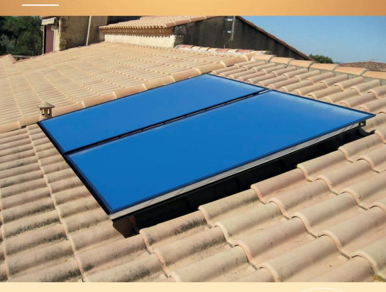
The individual solar water heater consists of one or more collectors, a storage tank and a regulation. The number of the collectors depends on the geographical area and the number of people living in the home. The storage tank can be supplied with back-up energy through an electric resistance, a heat pump or other boilers (gas, oil, wood).
